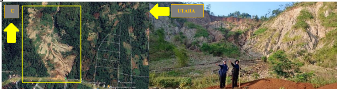
(Figure 1. Landslide Area)
