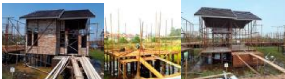
Figure 2. Frame Construction of Houses
