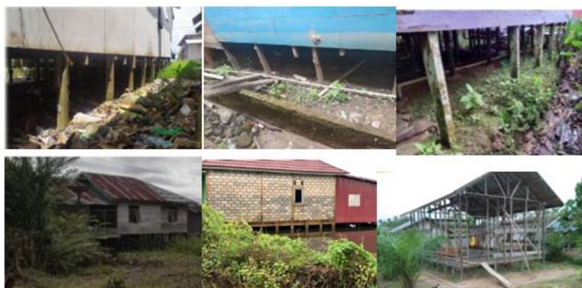
Figure 12. Foundation for Kotabaru, Kandangan, and Amuntai Areas
