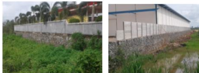
Figure 14. Use of Foundation on Soft Soil
