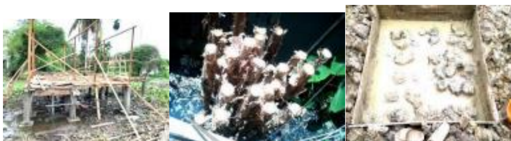
Figure 3. Use of Concrete Plate Foundation
