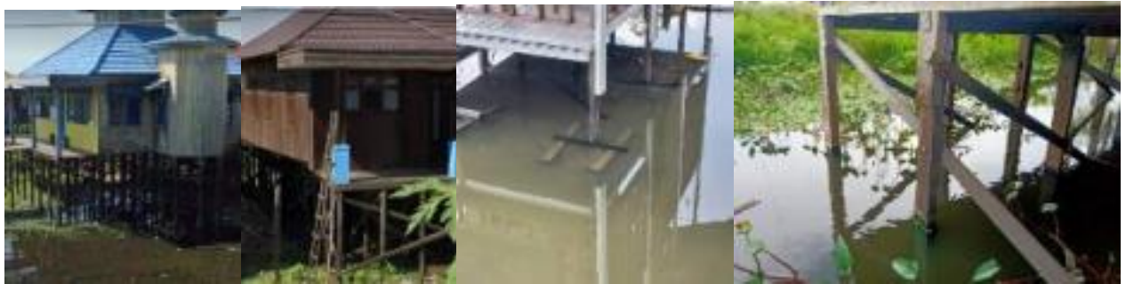
Figure 4. Wooden Pile Foundation in Banjarmasin
