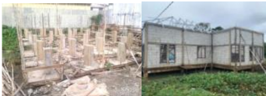
Figure 5. Concrete Foundation in Banjarmasin
