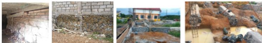
Figure 8. Amuntai Area Foundation
