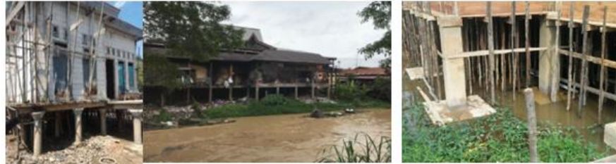
Figure 13. Foundation of Kotabaru, Kandangan, and Amuntai Areas
