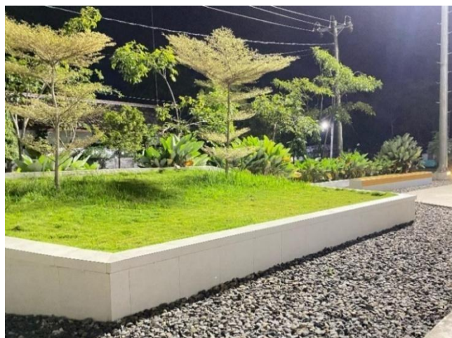
Gambar 11. Retaining Wall Taman
